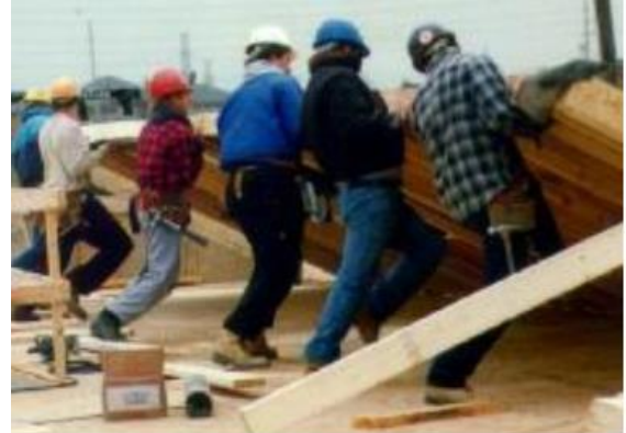
Manual wall lifting
