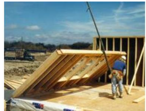
Lifting wall with a hydraulic
