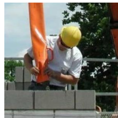
Filling the blocks
