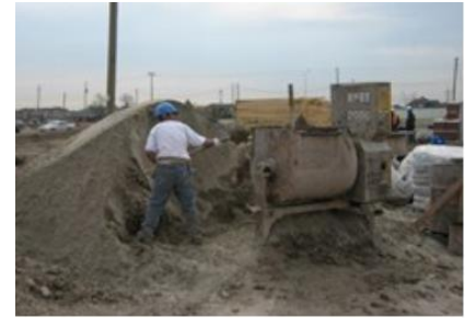
Traditional method of shovelling sand into a mixer
