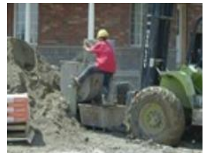
Traditional method of manually dumping the product from the mixer
