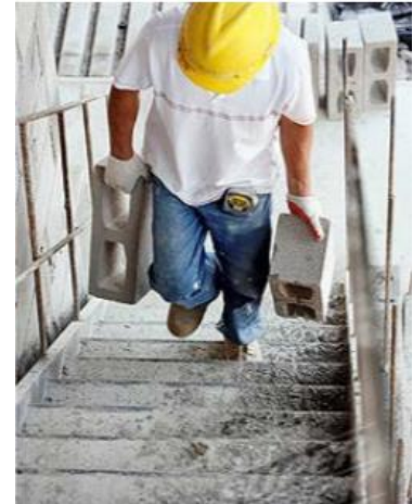
Manually transporting materials up the stairs
