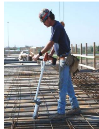
Rebar-tying tool with coiled spring wire
