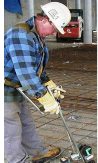
Rebar-tying tool with coiled spring wire
