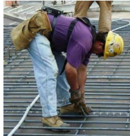
Tying rebar by hand
