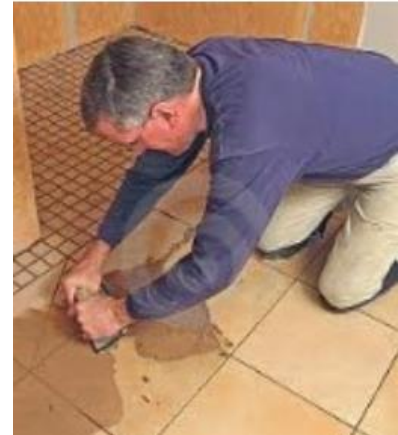
Kneeling on floor while grouting tile
