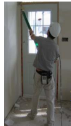
Finishing drywall using pneumatic drywall finishing system
