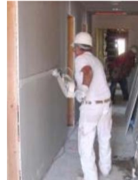
Finishing drywall using a traditional mudbox
